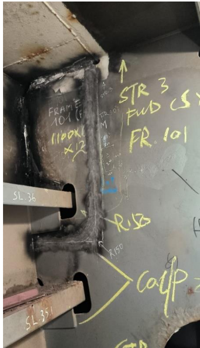
NEW STEEL INSERTION IN PROGRESS
